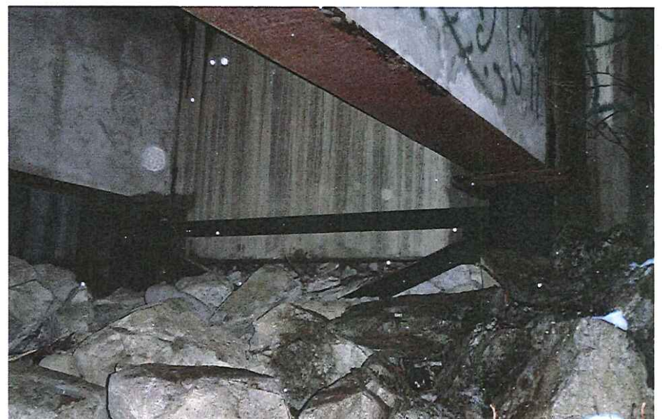
CK-2035 Abutment Right Bank #2
