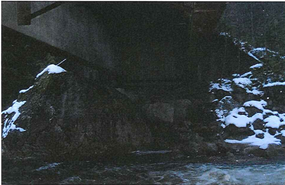
CK-2035 Abutment Right Bank
