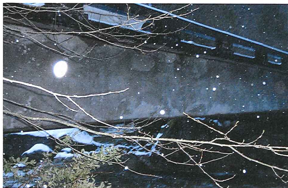
CK-2035 Crossing Upstream
