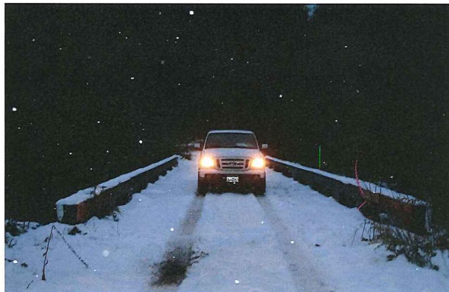
CK-2035 Approach Right Bank
