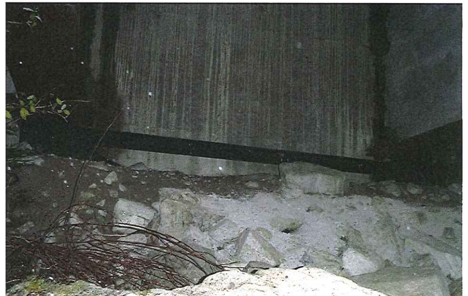
CK-2035 Abutment Left Bank
